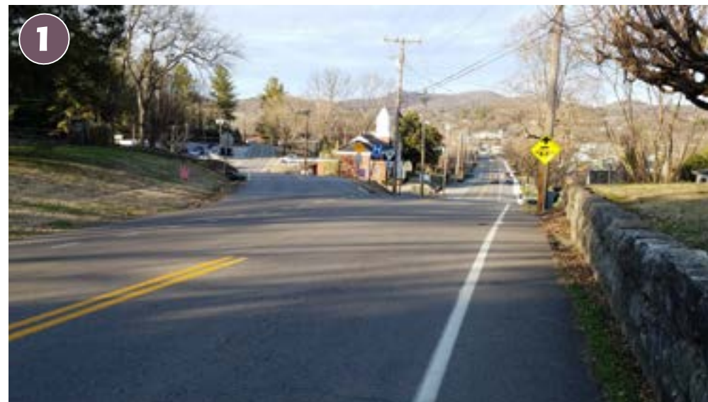
The intersection of River and Church Street has historically been a conflict point due to sight distance restrictions, poor signage, and lack of pedestrian facilities.
